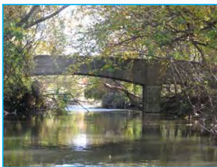
11:55 am Bridge in Eloise property
