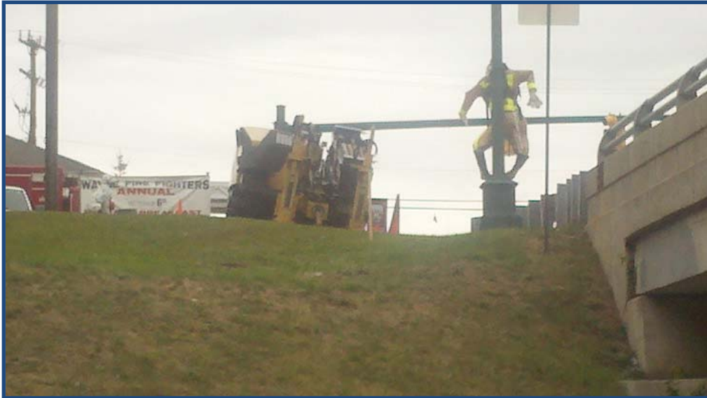
Directional drill equipment mobilized on the north bank, upstream of the bridge
