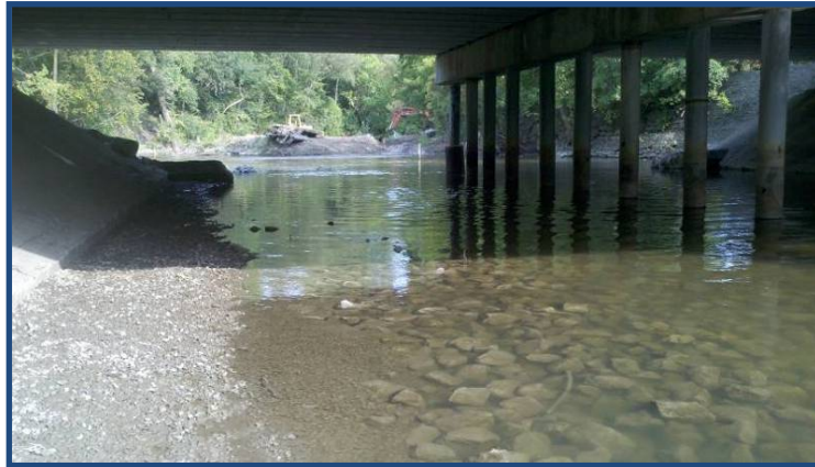
North half of riffle under the bridge, view looking east. Note smaller stone near the bridge abutment and larger rock in the stream channel. The smaller stone will eventually be covered with larger rock that will slope up against the abutments
