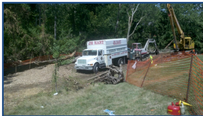
Clearing operations for west access route
