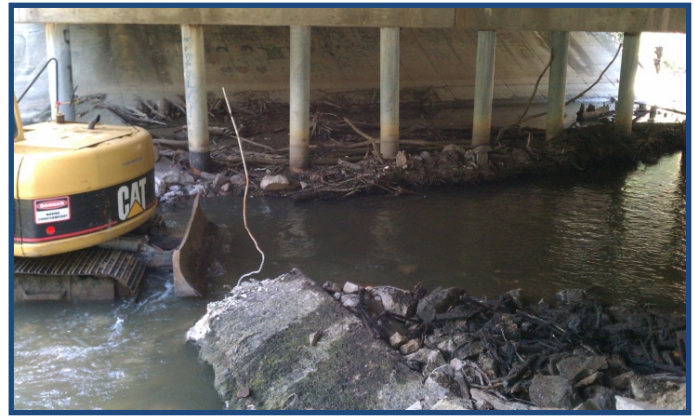
Notching of spillway
