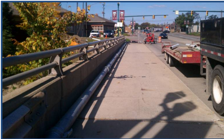
Diversion pipe used during sewer connection work
