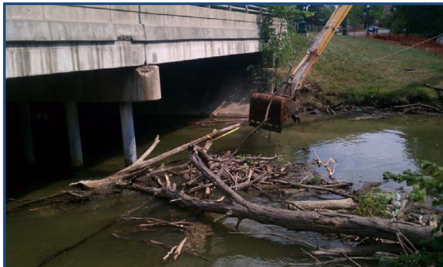
Log Jam Removal (Upstream Side of Wayne Road Bridge, view looking south)
