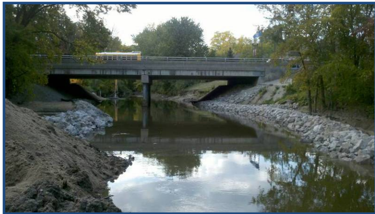
View looking west, note sand backfill behind a portion of the stone toe
