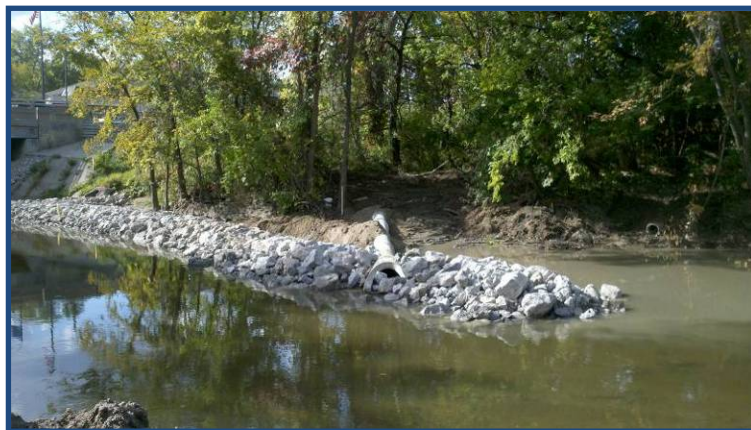
Storm sewer outfall at north bank downstream of the bridge
