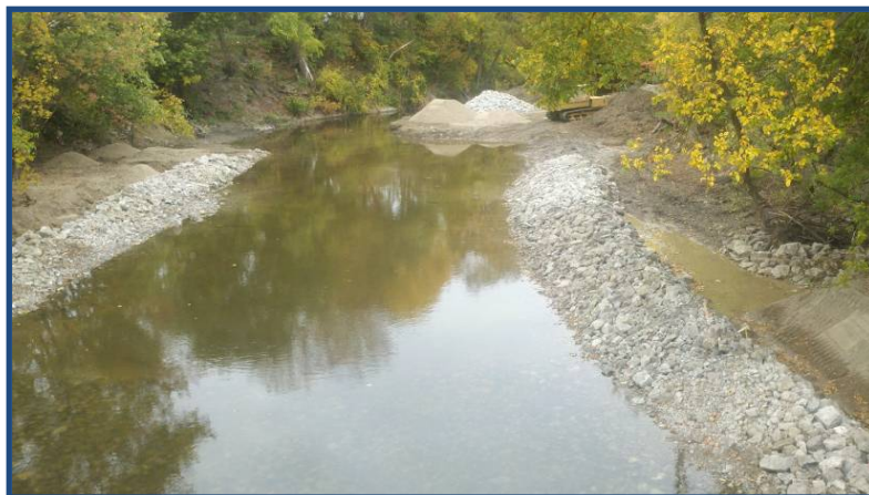
October 5, 2012: View from bridge looking downstream (east). Note: portion of rock placed and sand backfill.
